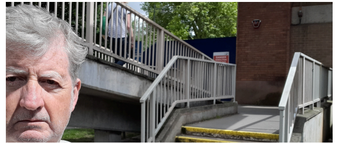
I've been promised a new, better ramp to Frankwell footbridge
